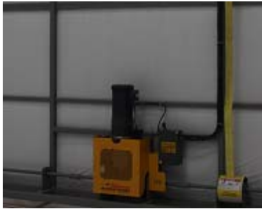
Motor mounted on the lower portion of the door.
