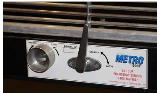
Interior view: The firefighter will have to first unlock the bolt, then unlatch the gate to lift.
