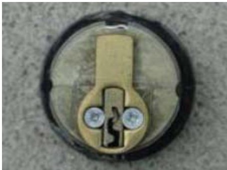
Lock Cylinder Removed
