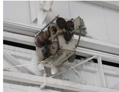
Motor mounted to the upper portion of the door.
