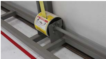
Motor turns a spindle the wraps the strap causing the door to lower and raise.
