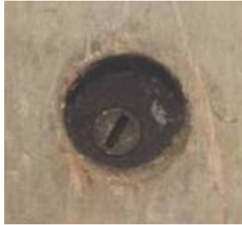
Lock cylinder removed
