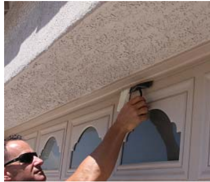
A wedge and/or inflatable bag create a gap between the door and jamb
