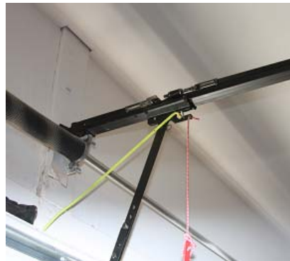
The rod or Slim Jim is hooked on the release latch and pulled downward
