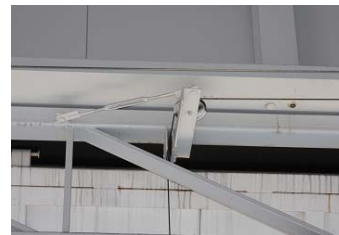
Motor turns a spool causing the wire to pull up or down on the lower portion of the door.
