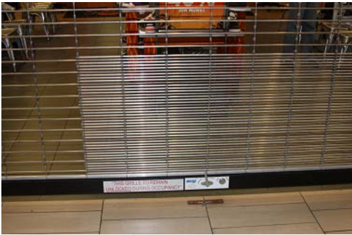
Exterior view: small section can be cut out above the lock so the firefighter can reach in to unlock and unlatch
